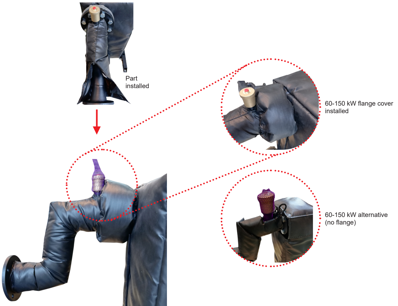
FIGURE 7 - Upper flow pipework installed (side view)
